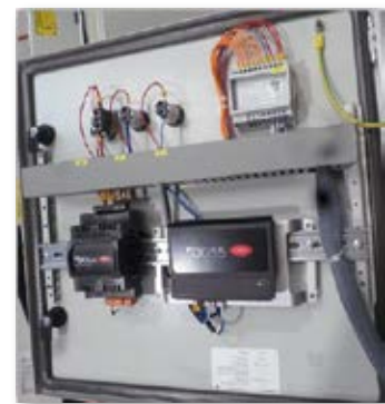
Fig. 1.a - Electrical panels with CAREL electronics
